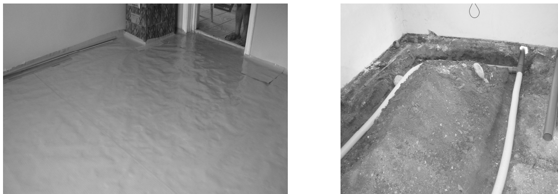
Fig. 6. Membrane installing above sub-slab depressurisation system
